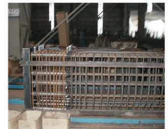
Assembling rebar cage for precast column
