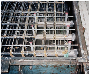
Precast wall before pouring concrete
