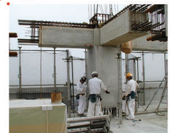
Erecting precast column
