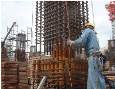
Slim Sleeve for connecting rebar cage
