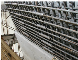
Bridge Pier Reinforcement
