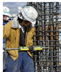
Injecting SS Mortar
