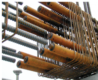
Sliding Slim Sleeve onto rebar
