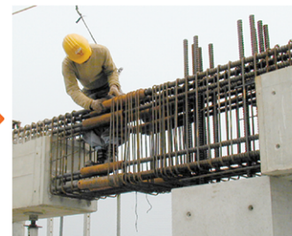
Placing stirrup
