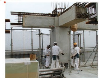
Erecting precast column
