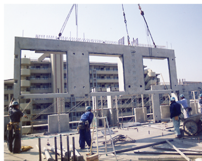
Precast concrete wall
