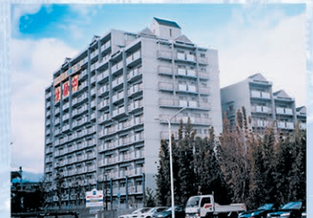
Damaged-free apartment buildings constructed with NMB Splice Sleeve in the epicenter at Kobe, Japan (Photographed on Feb. 17, 1995)
