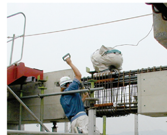
Injecting SS Mortar
