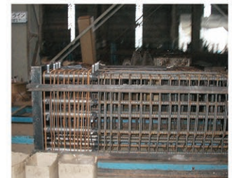
Assembling rebar cage for precast column
