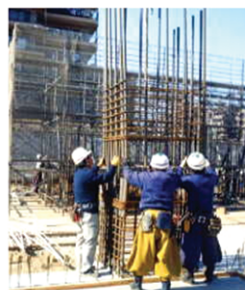
Lowering upper rebar cage
