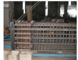
Assembling rebar cage for precast column
