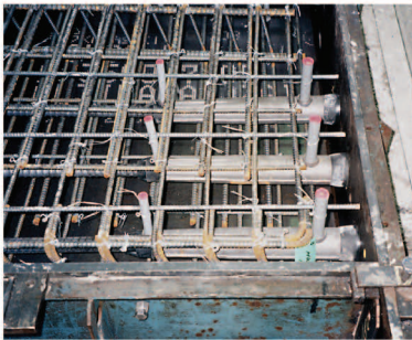
Precast wall before pouring concrete
