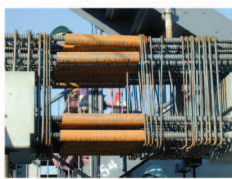
Slim Sleeve for connecting Precast beams
