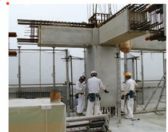
Erecting precast column
