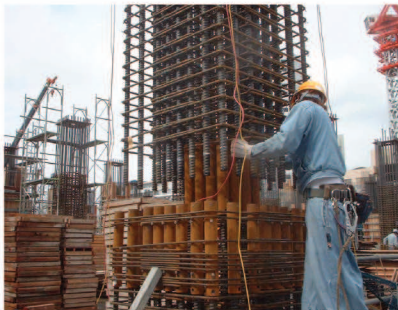
Slim Sleeve for connecting rebar cage
